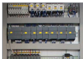
GESTIONE MACCHINA PLC SIEMENS MACHINE CONTROLLED BY PLC SIEMENS
